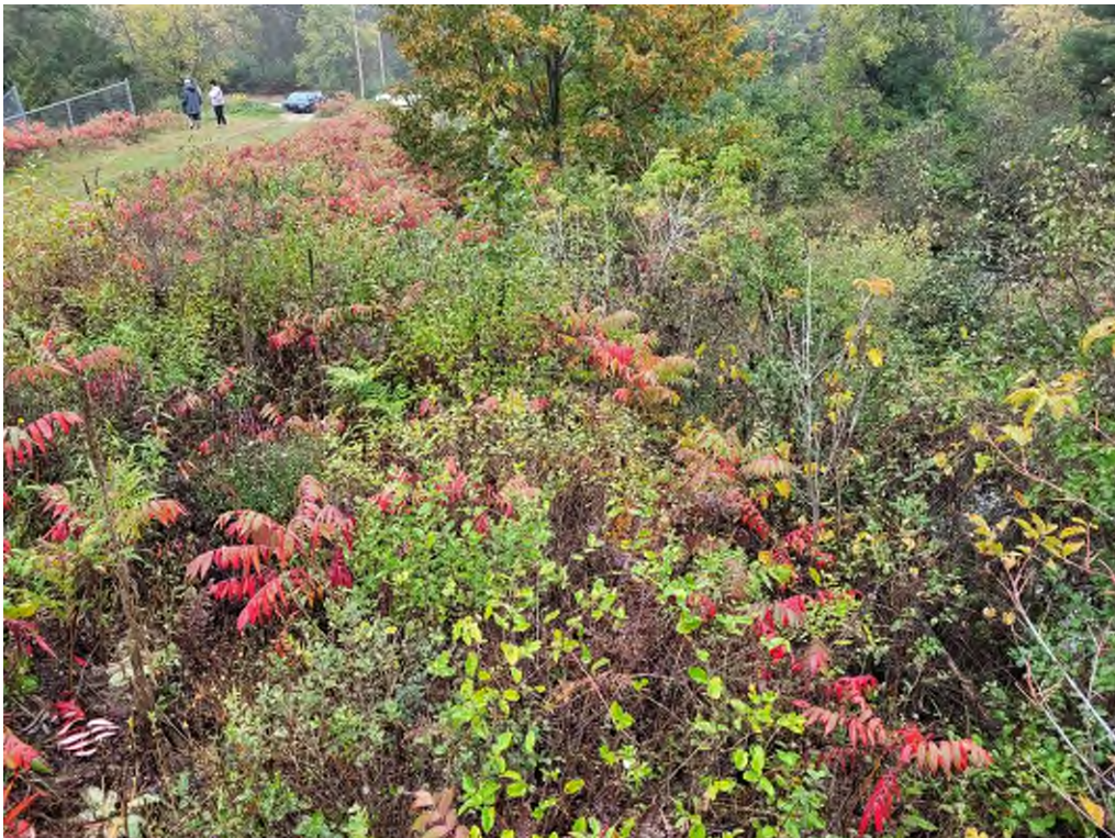
Photo #6 – Downstream slope looking left
