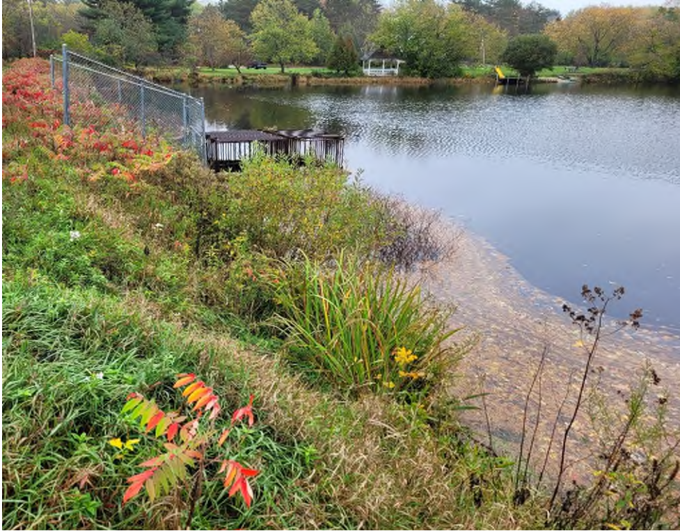
Photo #1 – Upstream slope looking right from left abutment
