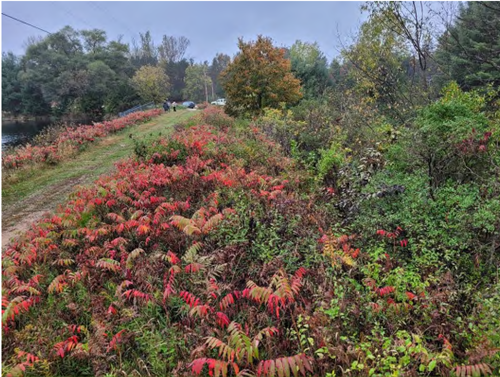
Photo #5 – Downstream slope looking left from right abutment
