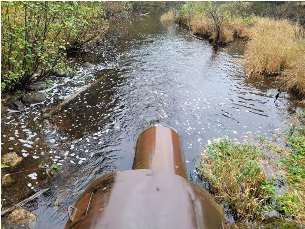
Photo #8 – Primary spillway outlet looking downstream
