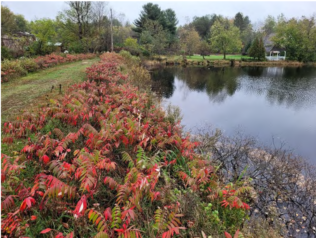
Photo #2 – Upstream slope looking right
