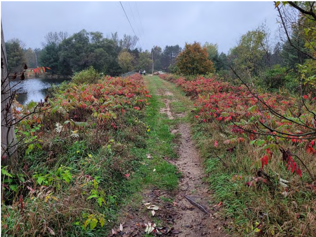
Photo #4 – Dam crest looking left from right abutment (low area)
