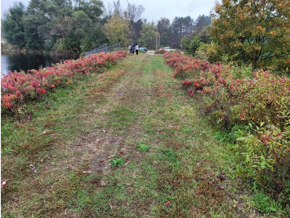
Photo #3 – Dam crest looking left
