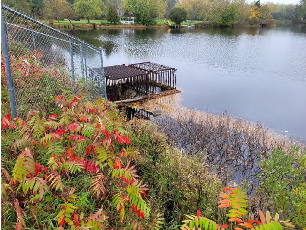
Photo #7 – Primary spillway looking upstream
